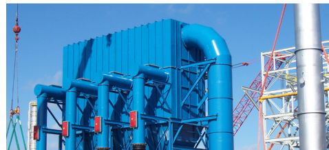
Dust Collectors provide high-efficiency particulate capture to control cement dust at critical points throughout the process.
